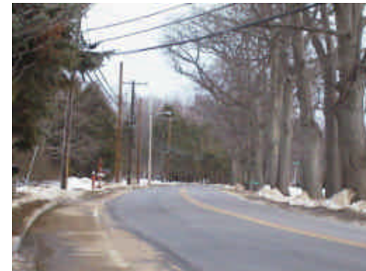
Dennett Road, Kittery, improved
