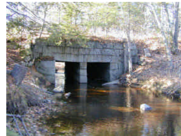
Double Box Culvert, Lovers Brook, South Berwick
