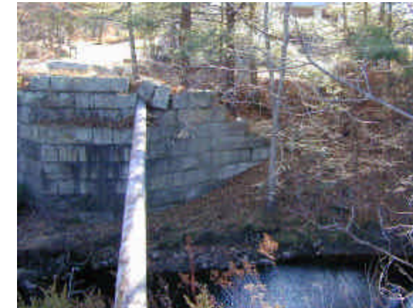
Missing Bridge at the Great Works River
