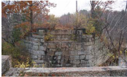
Looking north across Nonesuch River
