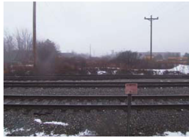
Guilford Rail Line, looking north
