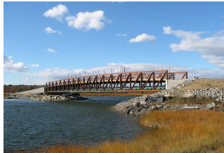
Where we've been ... the Scarborough Marsh Bridge just prior to opening in 2004.
