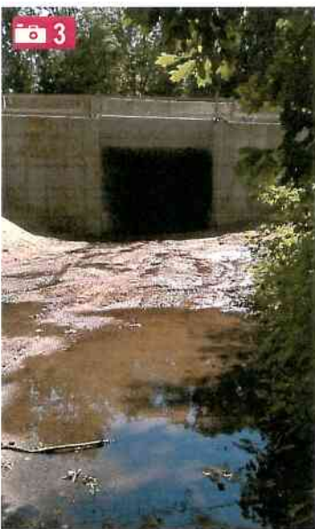
Photo 3 At Route 109 Current construction of trail underpass.
