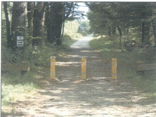
Example of collapsible bollards used on Scarborough trail section
