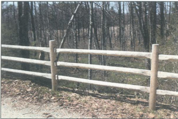
Example of cedar rail fencing used on Scarborough trail section.
