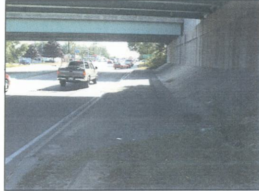
B2: Trail section, looking south, Passing under I-195 overpass
