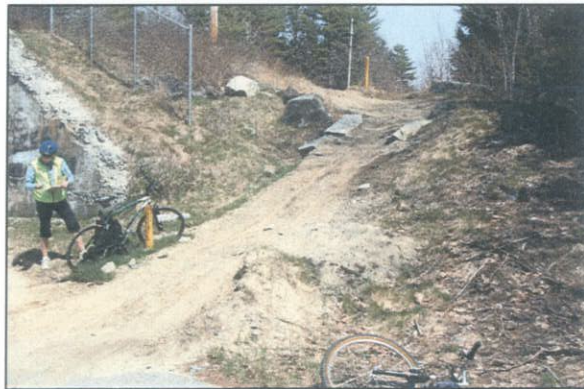
F5: Example of steep sections of trail that may require regrading, ramps and railings
