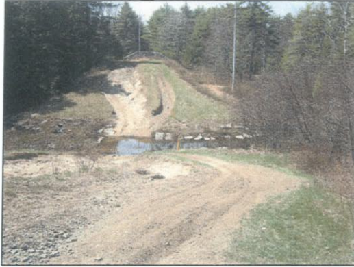
F6: Trail section, looking south, at Mill Brook stream crossing
