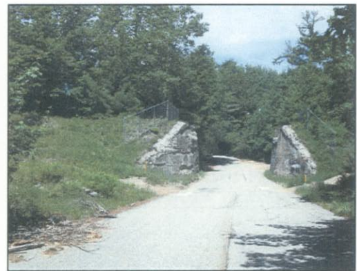
F4: Old Cascade Road crossing bridge abutments
