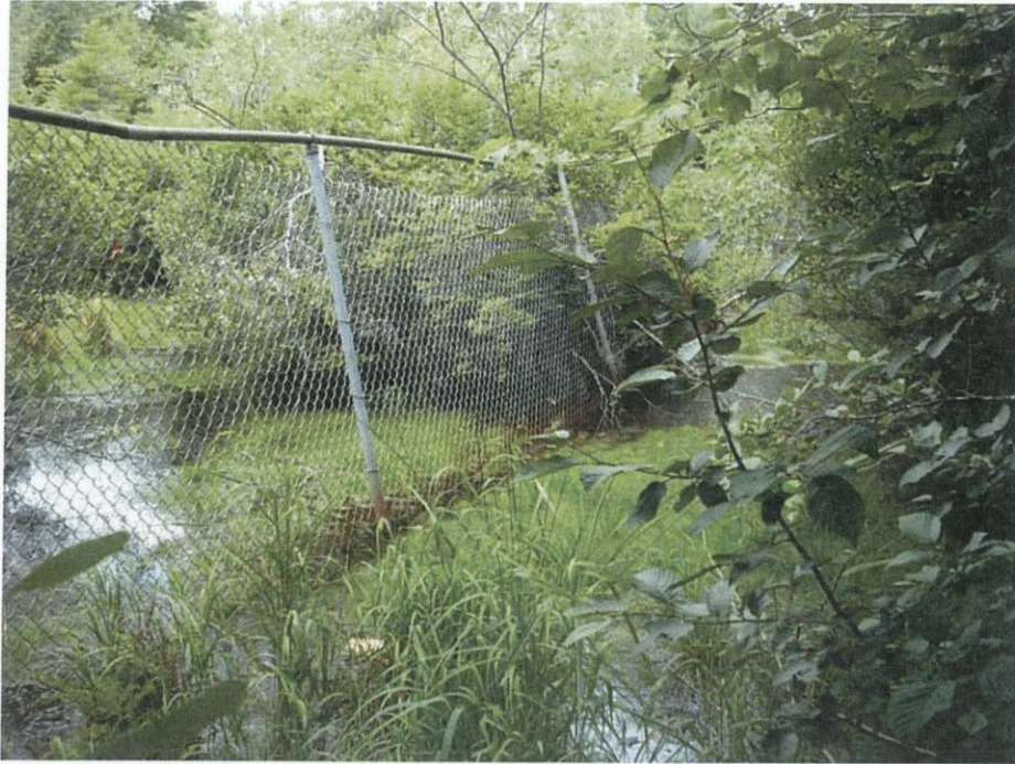
9- Facing south at large scrub/shrub wetland bordering south side of I-195
