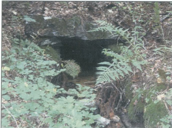
Outlet looking northwest
