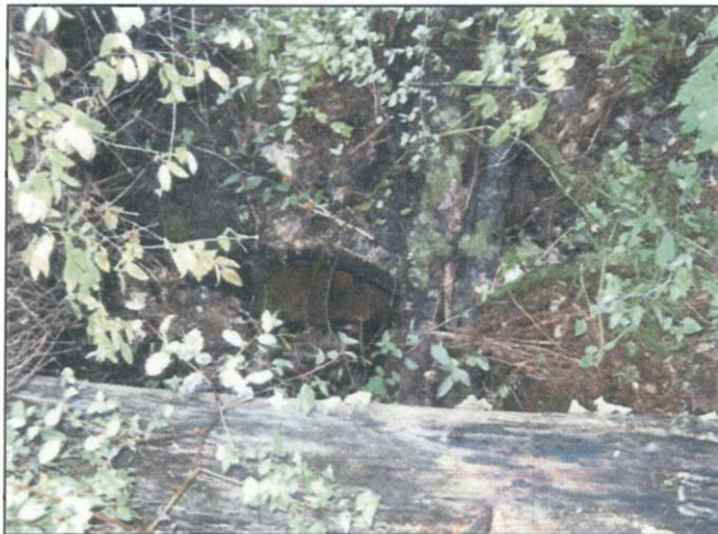
Inlet looking east
