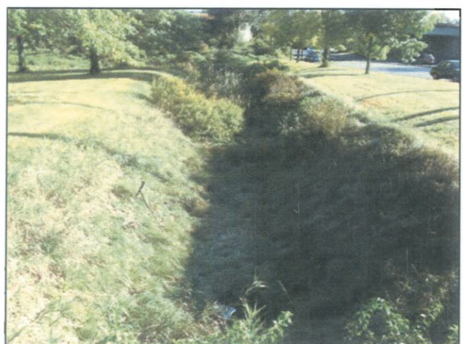
Outlet outfall to pond looking northeast
