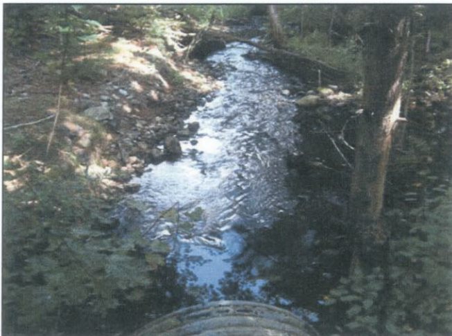
Outlet outfall looking north
