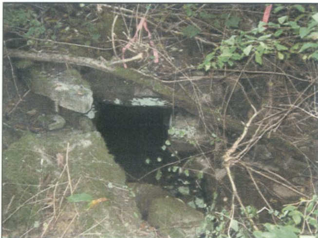
Outlet looking northwest
