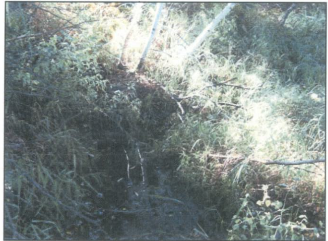
Inlet ditch looking southeast
