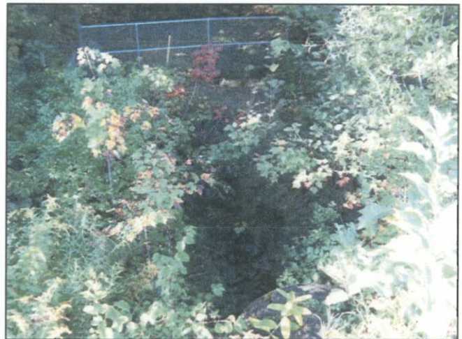
Inlet ditch looking west
