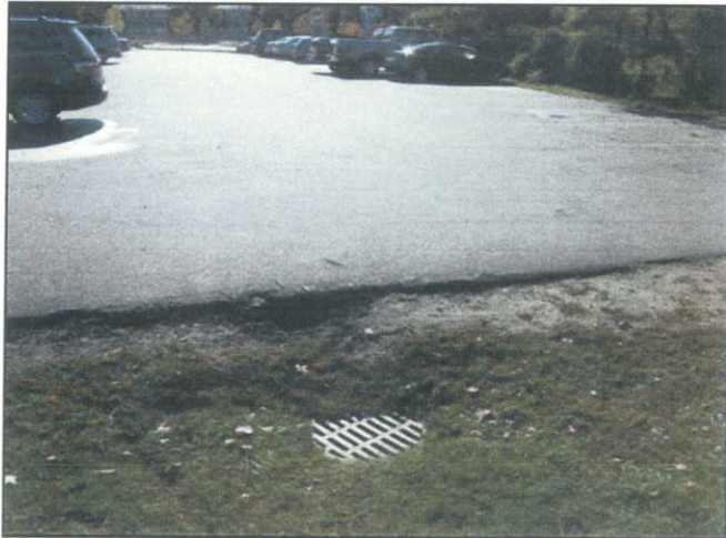
Catch basin inlet looking southeast
