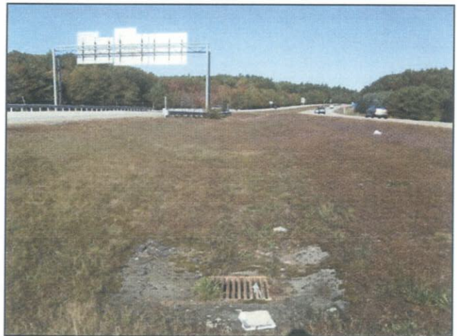
Catch basin inlet looking northwest
