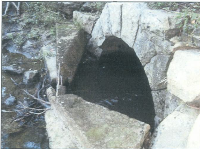
Inlet looking east
