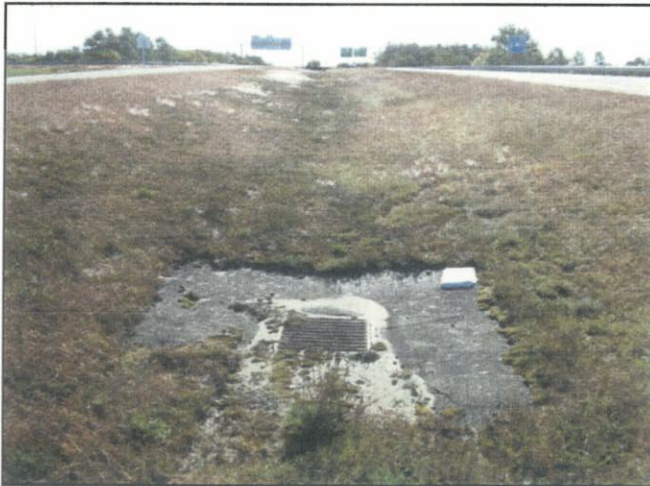
Catch basin inlet looking southeast
