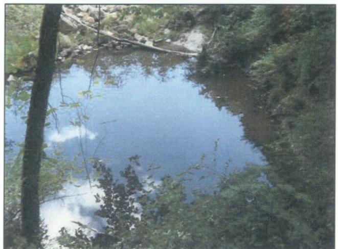
Outlet outfall looking southeast
