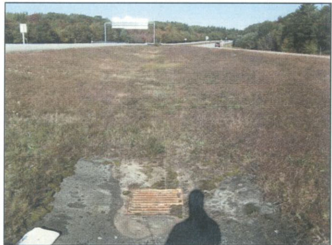
Catch basin inlet looking northwest
