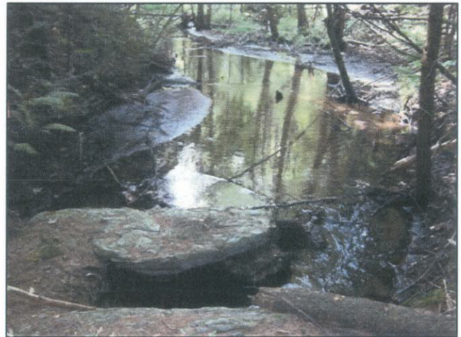
Inlet looking south
