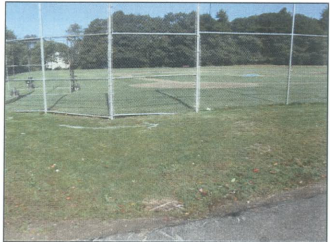
Catch basin inlet looking northwest
