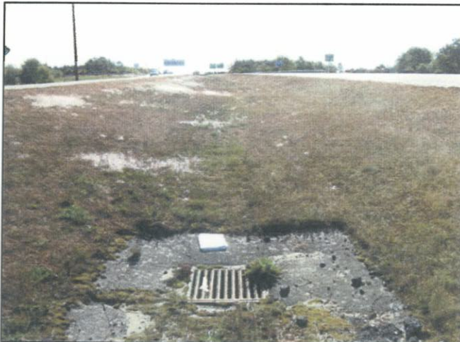
Catch basin inlet looking southeast
