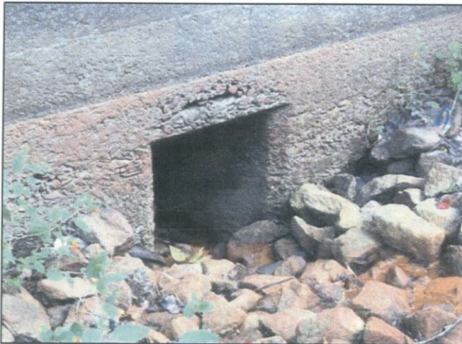
Inlet looking south
