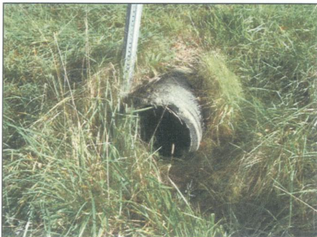
Outlet looking northeast
