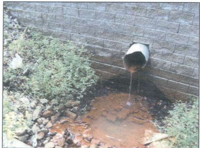
Seacoast RV site outfall looking northwest
