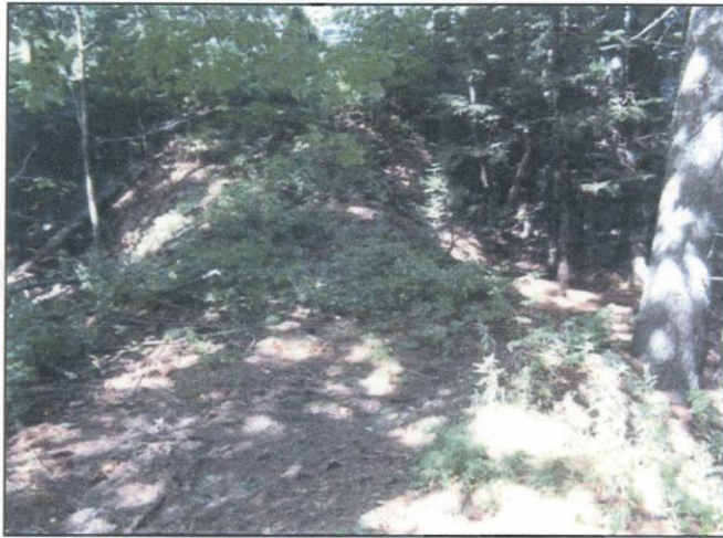
Access to abutting residence over culvert looking northwest from existing trail
