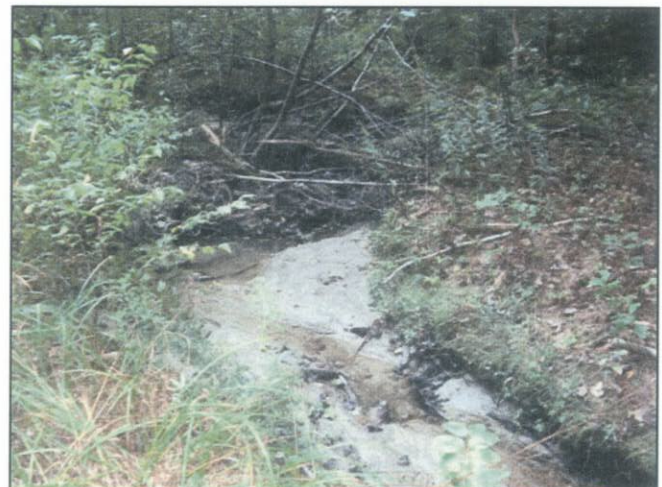
Outlet outfall looking southeast
