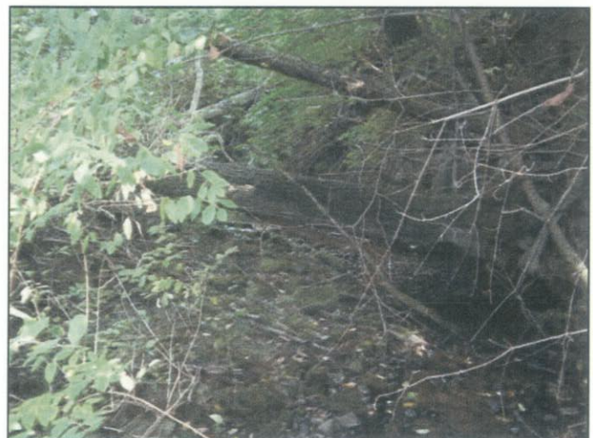
Outlet outfall looking southeast
