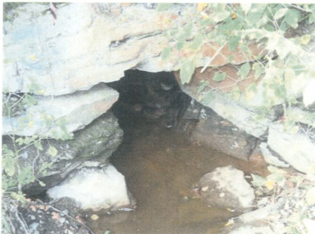
Outlet looking north
