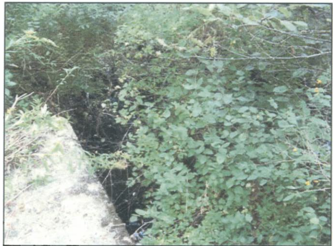
Inlet ditch looking west
