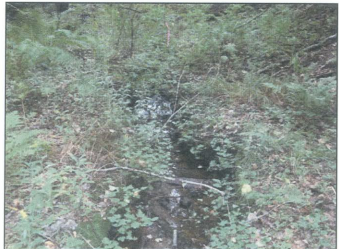
Outlet outfall looking southeast
