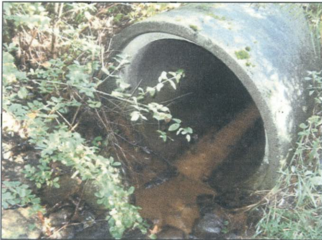
Inlet looking east
