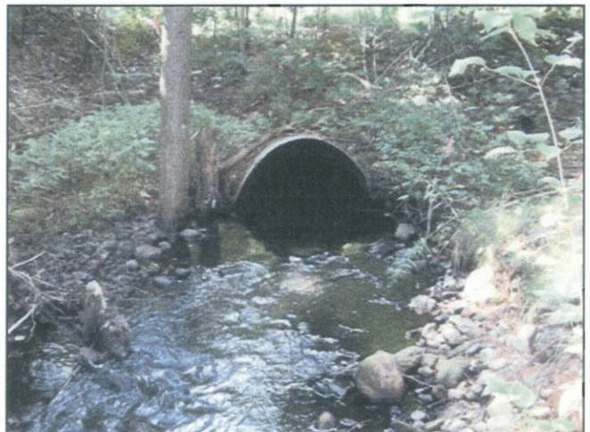
Outlet looking south
