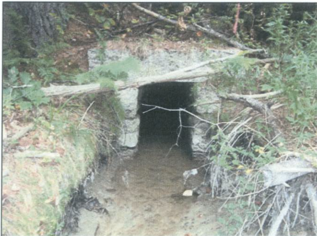
Outlet looking northwest
