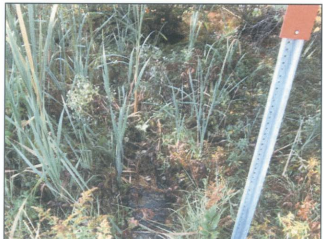
Outlet outfall looking southwest
