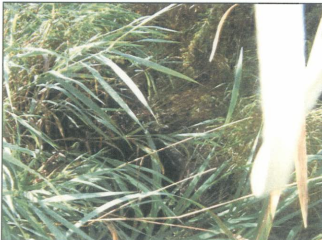
Outlet looking southeast
