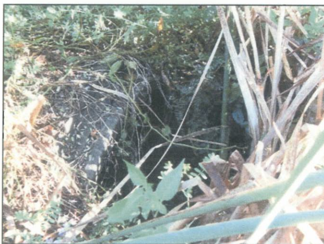
Outlet looking northwest
