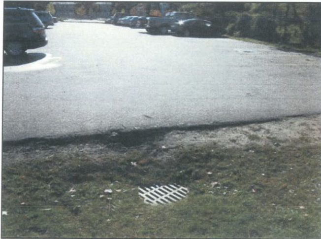
Catch basin inlet looking southeast
