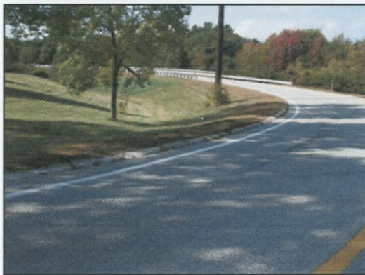
West view of off-ramp
