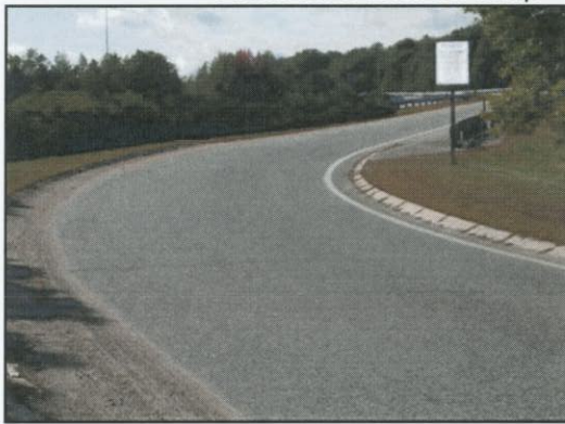
West view of on-ramp
